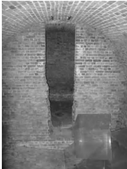
Figure 5.1 The ice house at Syon Park, Brentford, south-west London. This was constructed in the 1820s by order of the third Duke of Northumberland to replace earlier seventeenth/eighteenth century structures. The ice was tipped into the storage chamber via the roof and packed in straw. The store had a sump draining to waste via a sloping floor. Access to the ice house was via an ‘airlock’ of two doors. The ice house was not dug vertically downwards to any great extent but was subsequently covered by soil to form a landscaped mound. The ice, being collected from lakes and the River Thames, was impure and not consumed directly. It was, however, used by the aristocrats to cool drinks and produce sorbets and ice creams (by adding salt to form a freezing mixture). Photo by David Banks.
