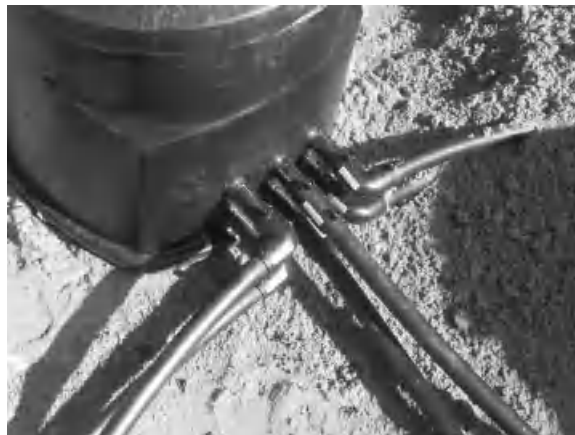
Figure 9.7 A prefabricated manifold chamber, showing three ground-loop circuits connected in parallel, using electrofusion couplings. Photograph reproduced by kind permission of Water and Energy Field Services Ltd.
