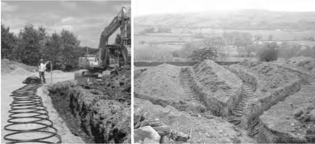
Figure 7.15 Two photos showing the installation of slinky-based horizontal closed-loop systems in trenches. The right-hand photo shows the installation of slinky-based horizontal closed loops in trenches on a hillside, spaced at about 4–5 m from each other. Photos reproduced by kind permission of Geowarmth Heat Pumps Ltd.
