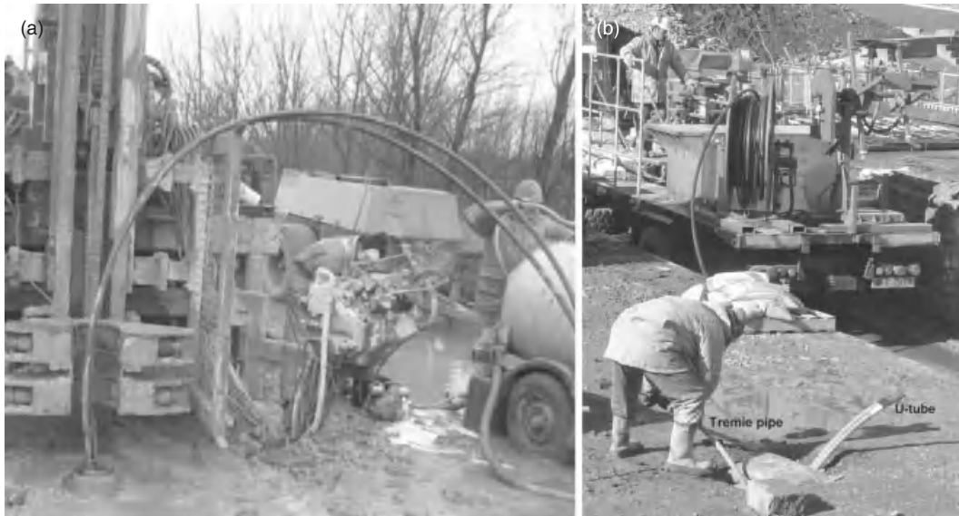
Figure 7.19 (a) Persuading a U-tube to descend a fluid-filled borehole can be trickier than it sounds, and it can also be messy. (b) Pumping grout into a closed-loop borehole. The reel of the tremie pipe and the tank containing the grout are mounted on the lorry. Photos reproduced by kind permission of Geowarmth Heat Pumps Ltd.
