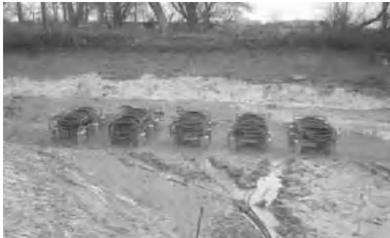
Figure 12.5 Five pond mats (loose coils of polyethylene pipe, anchored to a steel frame) in the base of a newly constructed artificial lake in Yorkshire, UK, designed to support a heat pump installation of c. 22-kW peak output. Photo reproduced by permission of Geowarmth Heat Pumps Ltd.
