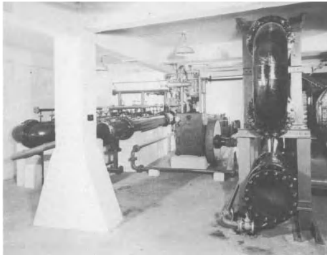
Figure 5.4 John Sumner's Norwich heat pump, from 1946 (see Box 5.3). Not so much a unit as a whole room! After Sumner (1976a).
