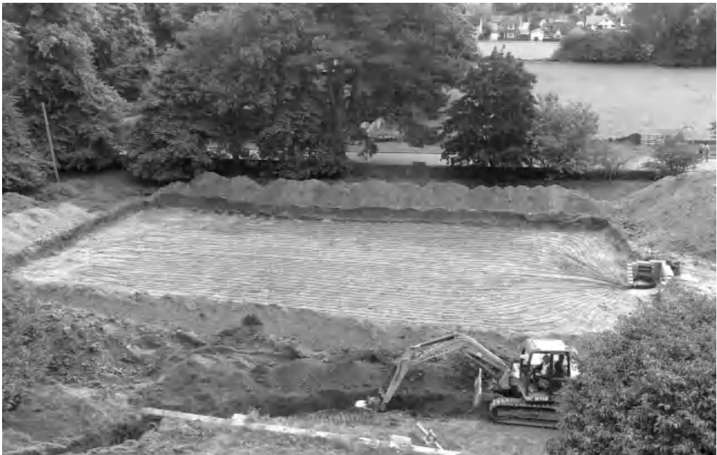
Figure 11.5 An array of horizontal pipework, comprising individual loops of single polyethene (PE) pipe returning to a manifold chamber (of the type shown in Figure 11.4c), being installed below a British field. The array is designed to support a heat pump installation of 15kW. Photo reproduced by kind permission of Geowarmth Heat Pumps Ltd.
