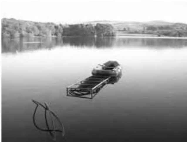
Figure 12.7 Coils for installation in a natural lake can be mounted in a steel frame, rowed out into the lake, filled and submerged. Photo reproduced by kind permission of Geowarmth Heat Pumps Ltd.
