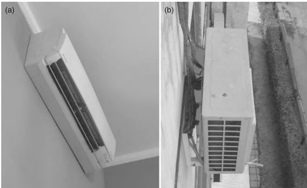
Figure 6.7 A split air conditioner, showing the interior (a) and exterior (b) units. Photos by Dave Banks.
